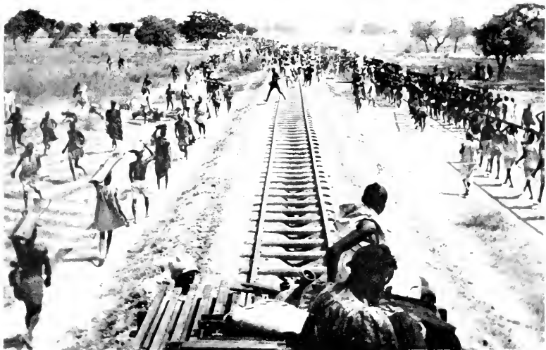
PLATE-LAYING ON THE NORTHERN NIGERIA RAILWAY.
